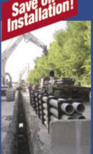
Assemble Conduit Above Trench-No Workers Below -Prevents Injuries and Deaths. Also Allows Digging a Narrower Trench for Less: Excavation, Concrete, Slurry, Backfill & Shoring.
